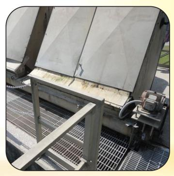
The Static Screen unit is a proven, reliable performer for liquid/solid separation in municipal and industrial applications, particularly for screening fibrous and nongreasy solids. There are no moving parts, motors, or complicated connections. The Static Screen is simple and economical to operate.
